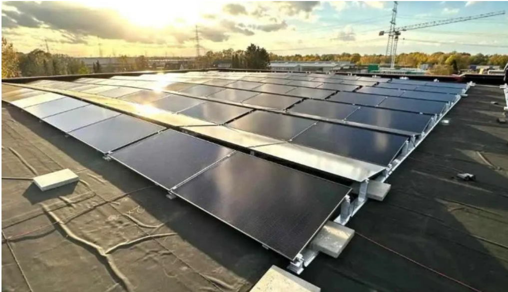
Jf montage photovoltaik montageservice bredstedt
